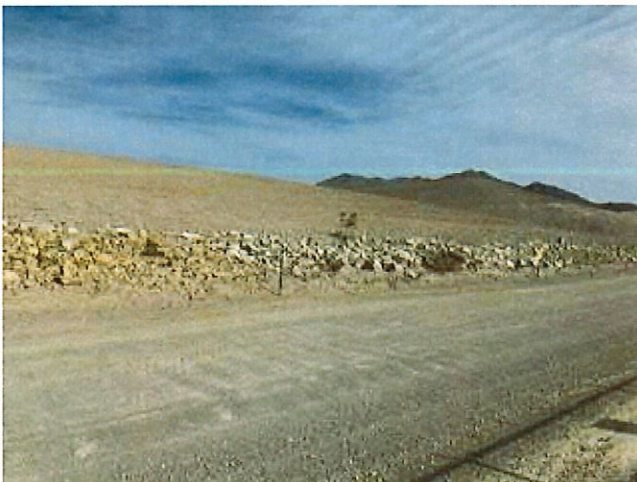
1 - Missing RAM sign on the South side.
