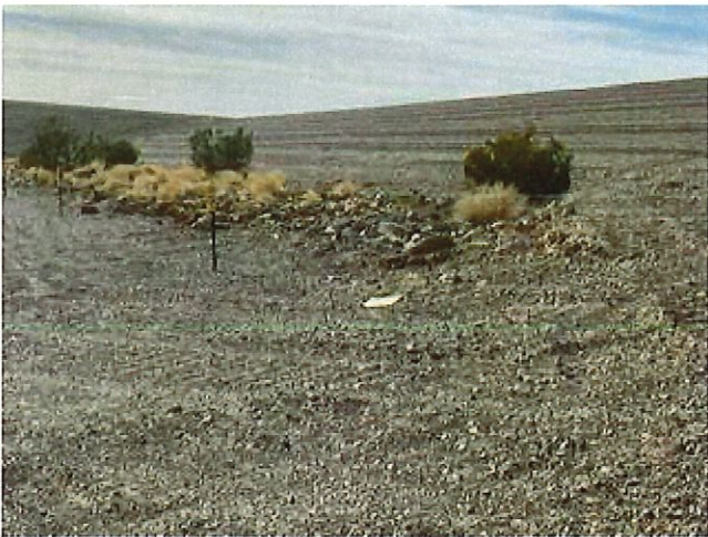
2 - Missing RAM sign on the NE Corner.
